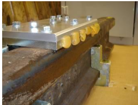
95lb Bull Head Check / Restraining Rail
